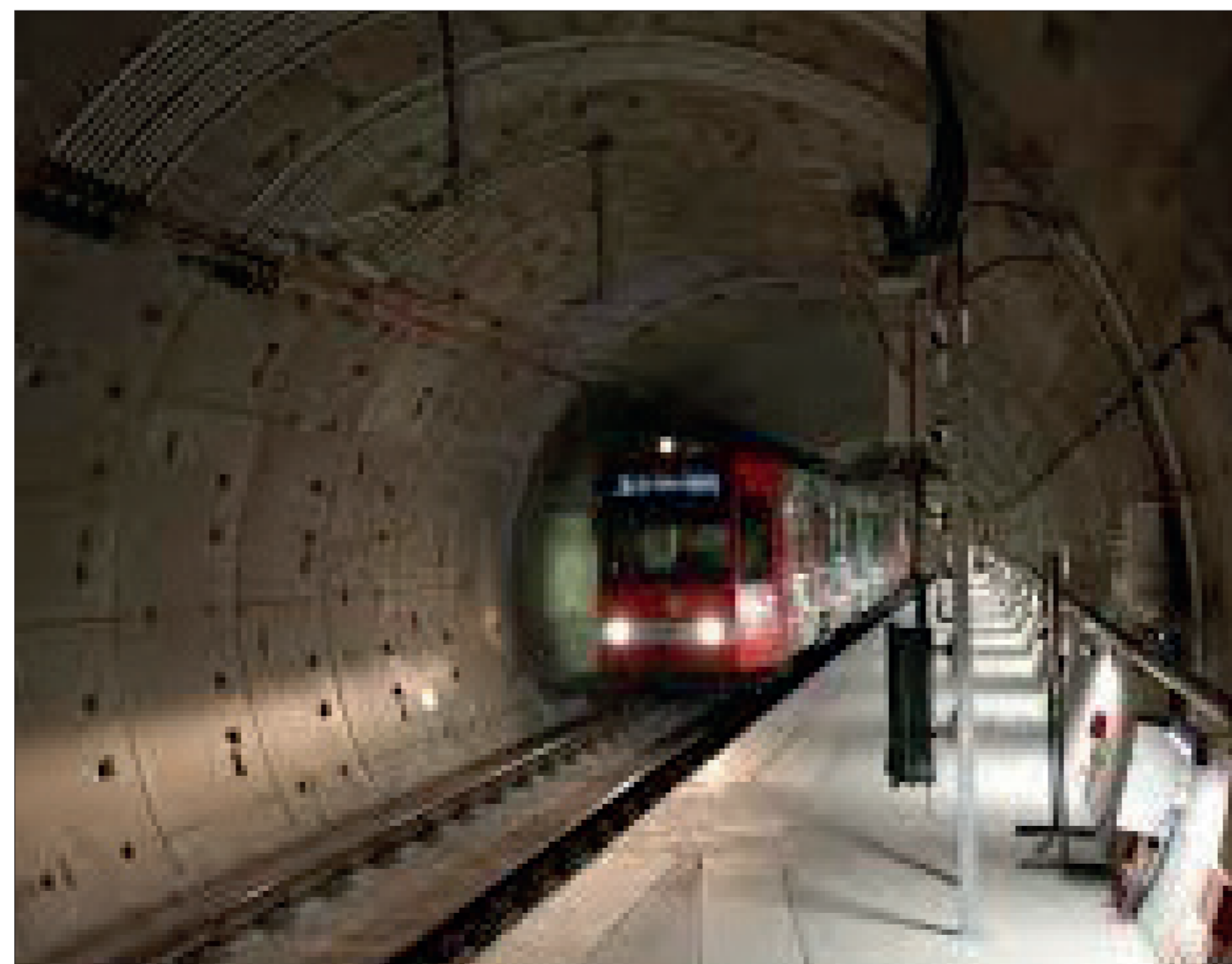
The tube transportation system can be implemented in already used tunnels by the KVB as they don't take up much space
