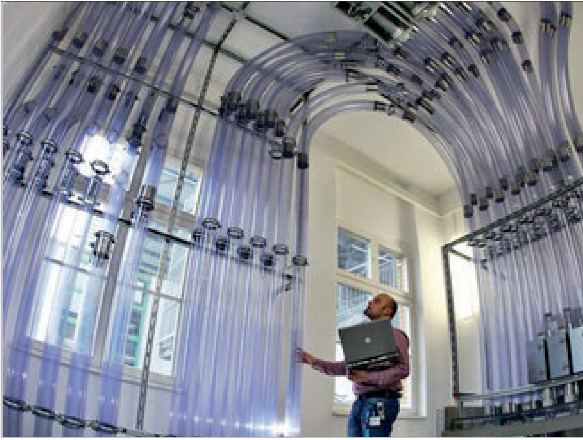
Tube stations to send and receive capsules. The destination can be determined by entering the destination's code on the device.
